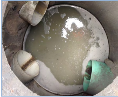
Suds found in a catch basin in St. Johnsbury which drains to the river, identified in an Illicit Discharge Detection & Elimination Study and corrected thru outreach
