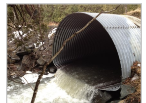
Culvert with no aquatic organism passage prepared for replacement in Danville, VT
