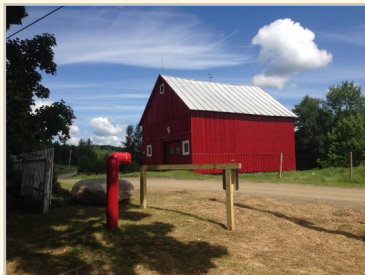
Dry hydrant installed in Enosburg
