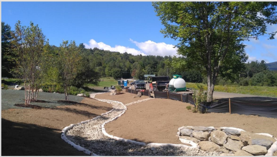
Implementation of a stormwater mitigation project at the Rumney Memorial School in Middlesex, installed by the Winooski Conservation District
